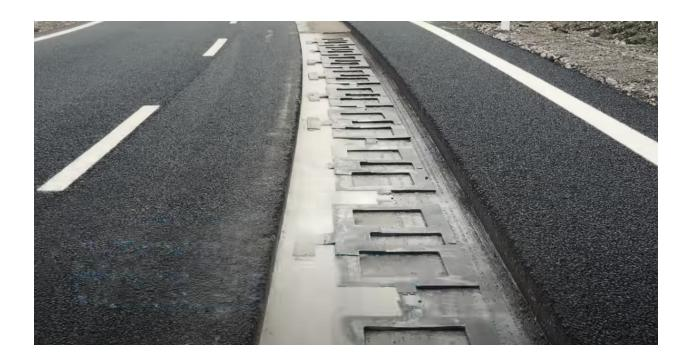
Transmission coils embedded in Stellantis's electric roadway.
